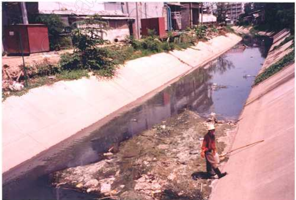
Figure 8. The Sewage Canal Site SC2
