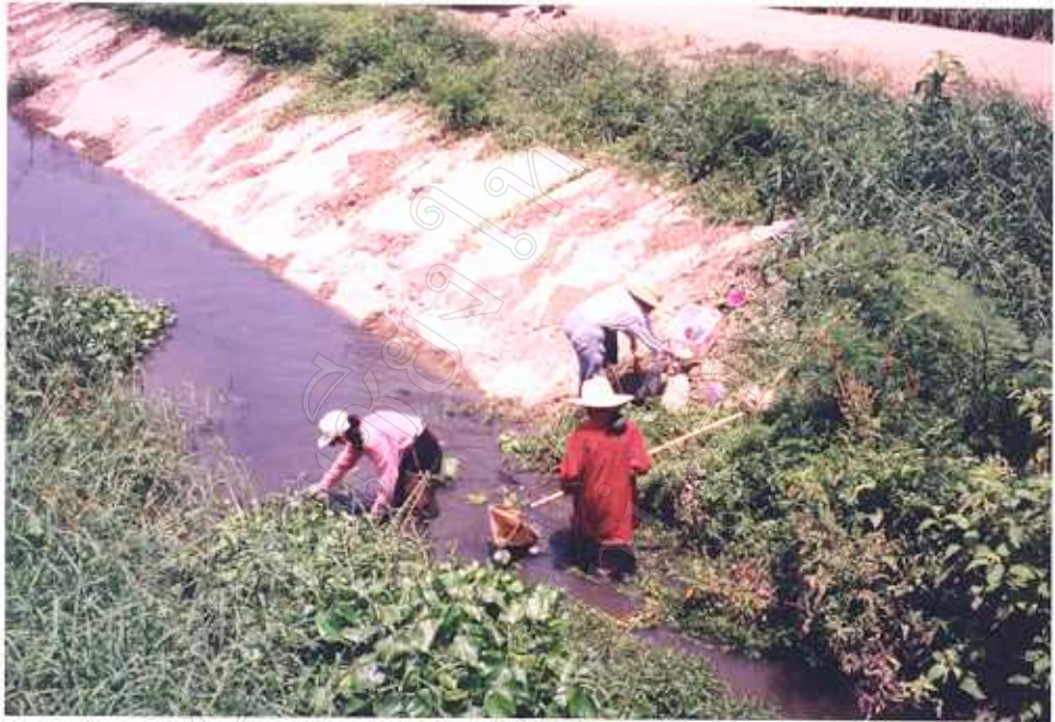
Figure 7. The Sewage Canal Site SC1
