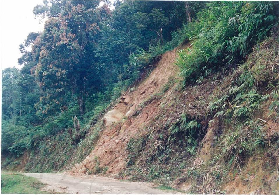
Figure 8. EGFX showing a landslide along the dirt road through Mae Kampong Village bordering a tea plantation (1050 m, 14 Nov. 1996).
