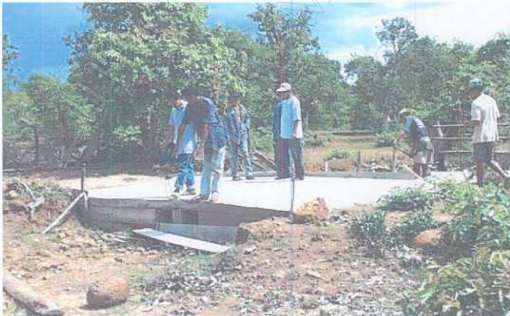
Appendix E Constructing a sluice gate at Nong Bua
