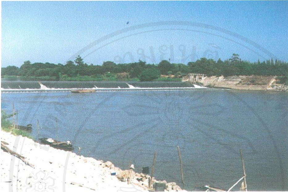
Figure 4. Wangpan Dam, Chom Thong District, Chiang Mai Province.
