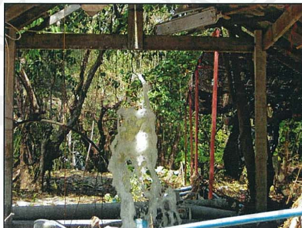
Figure 4.14 Photographs of Rehabilitating groundwater well (The Department of Groundwater Resources, 2005).
