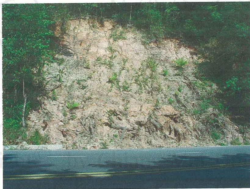
Figure 3.16 Picture of existing landslide (Landslide 8) in weathered gneiss before reaching Doi Suthep Temple.
