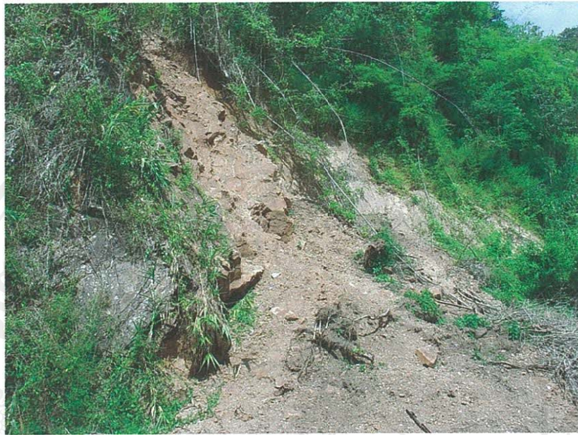
Figure 3.11 Picture of existing landslide (Landslide 3) in weathered gneiss on road leading to Ban Sam Lang
