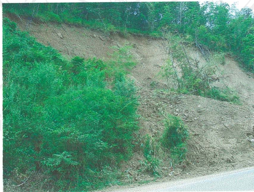
Figure 3.14 Picture of existing landslide (Landslide 6) in weathered shale on highway 1096 (Mae Rim-Samoeng highway)
