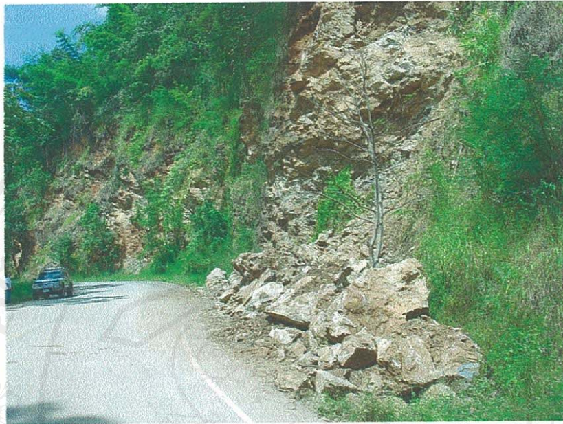
Figure 3.13 Picture of existing landslide (Landslide 5), a rock fall in limestone on highway 1096 (Mae Rim-Samoeng highway).
