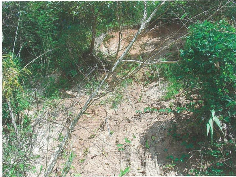
Figure 3.9 Picture of existing landslide (Landslide 1) in weathered gneiss on highway 1096 (Mae Rim-Samoeng highway)
