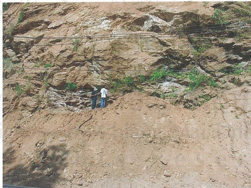
Figure 3.9 Picture of existing landslide (Landslide 1) in weathered gneiss on highway 1096 (Mae Rim-Samoeng highway)
