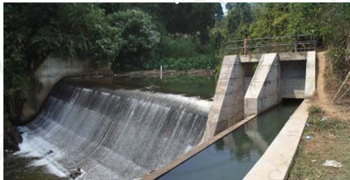
Figure 2.4 Intake weir of Nam Mong MHP in Luang Prabang province of Lao PDR.
