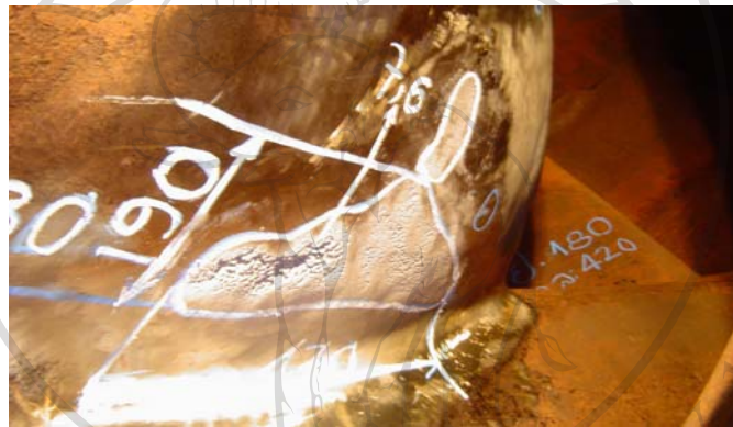
Figure 2.13 Cavitation of hydraulic turbine (Nam Ngum1 HPP).
