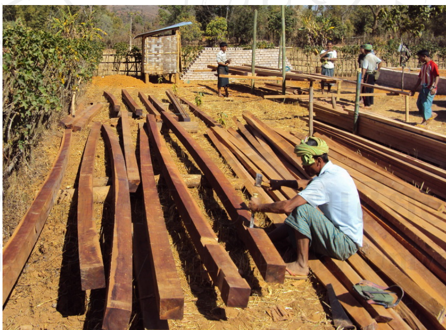
Figure 3.16: Daily Wage Workers Help with House Building Activities
