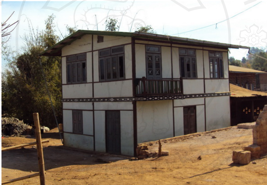
Figure 3.11: Concrete House of a ‘Better-off’ Household
