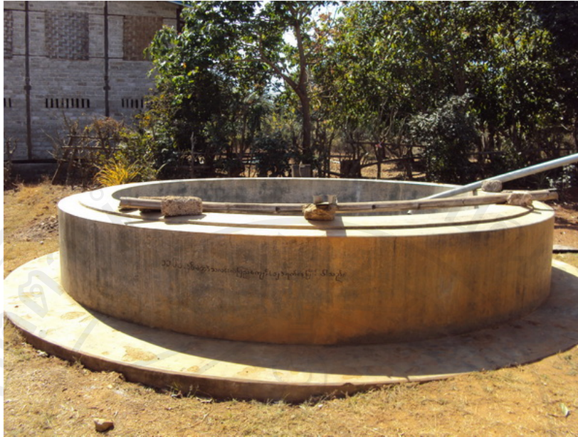
Figure 3.19: Concrete Tank for Collecting Rain Water
