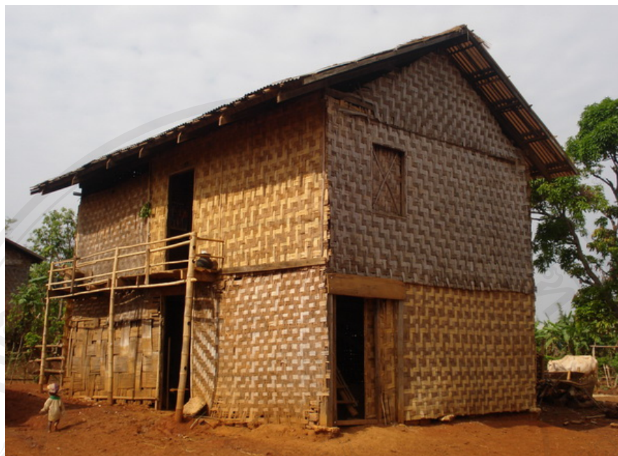
Figure 3.12: A Poor Family's Bamboo House
