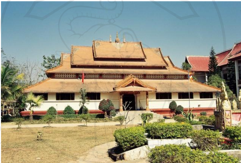
Figure 3.3: The old Vihaan of Wat Pajie, demolished at the end of 2008 (Image: Roger Casas)
