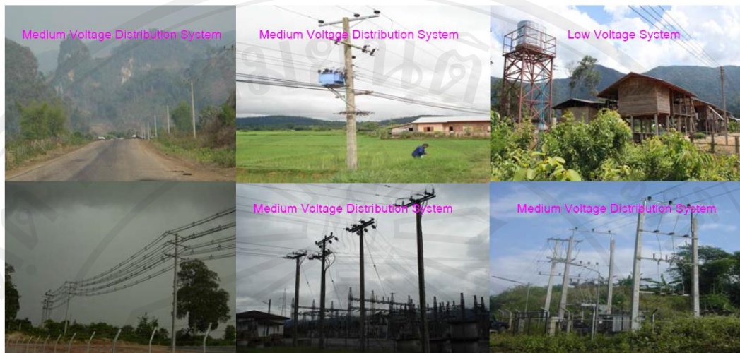
Figure 3.5 Distribution MV( 12.7kV, 22kV, 25kV, 34.5kV and 35kV and LV 0.4 kV
