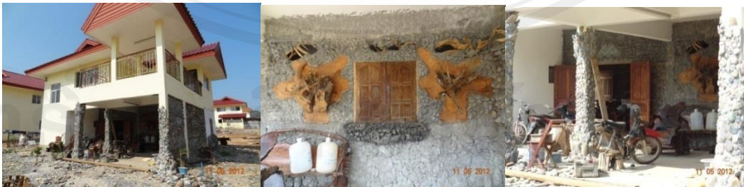
Figure 5.4: House Renovation since the Resettlement
