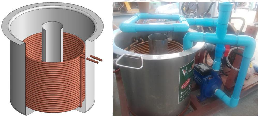
**Figure 3.6:** Water cooled condenser design and installation
