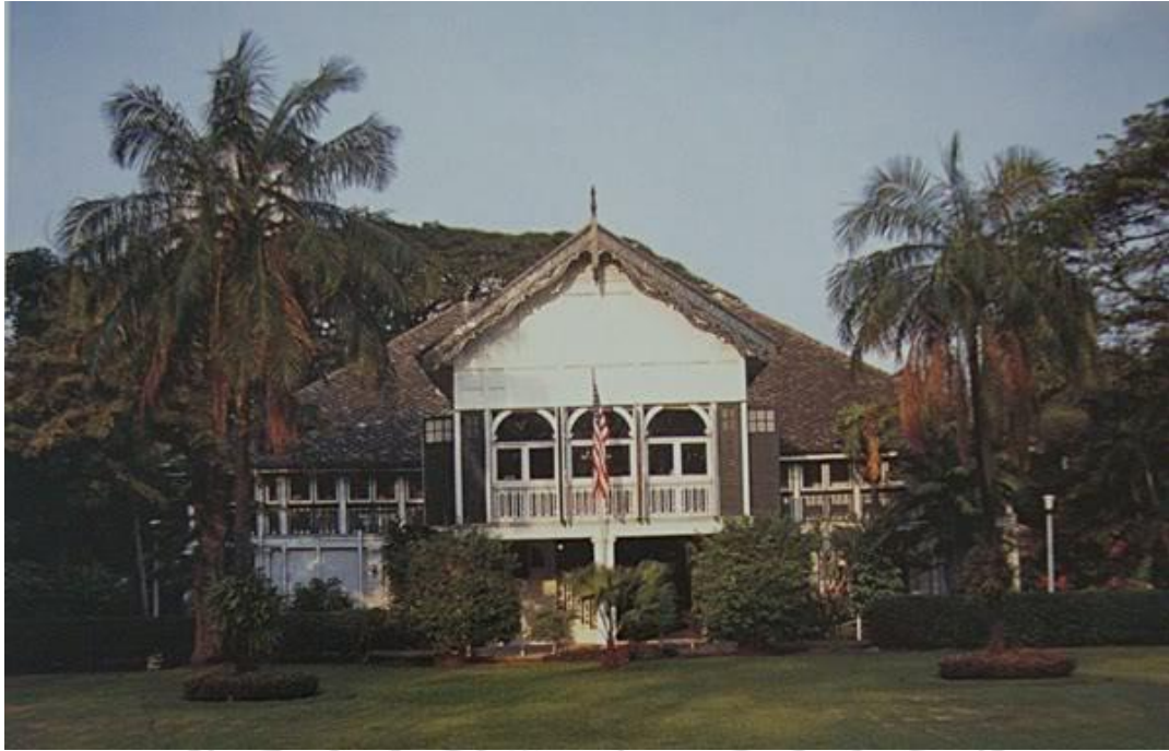
Figure 2.17 The American Embassy Residence is a Colonial house
