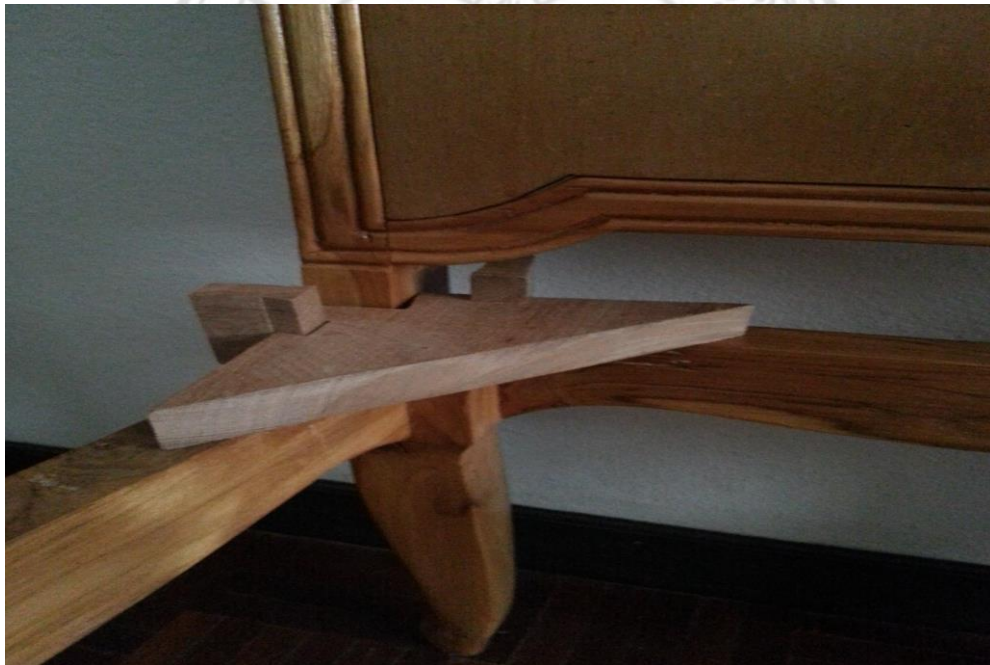
Figure 4.75 The using of Joint replacement by nail in the small area
