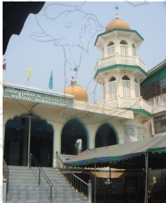
Figure 6.2: Nurul Islam Mosque after its second renovation (today)
