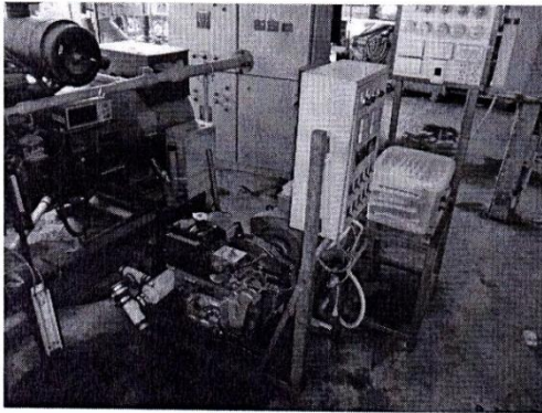
Fig. 2. Photograph of the small producer gas engine setup.
