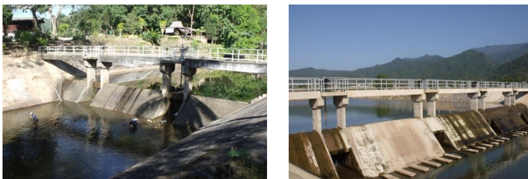
Figure 3.18 Two weirs blocking the Yang River before reaching TK Village, the old one constructed in the 1960s (left) and the latest one constructed in the 2010s (right)
