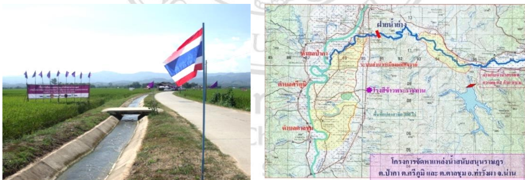
Figure 3.7 Restructuring the Yang River for supporting HRH Rice Mill, the infrastructure for field trials (left) and an official map showing the targeted rice paddy fields (right)
