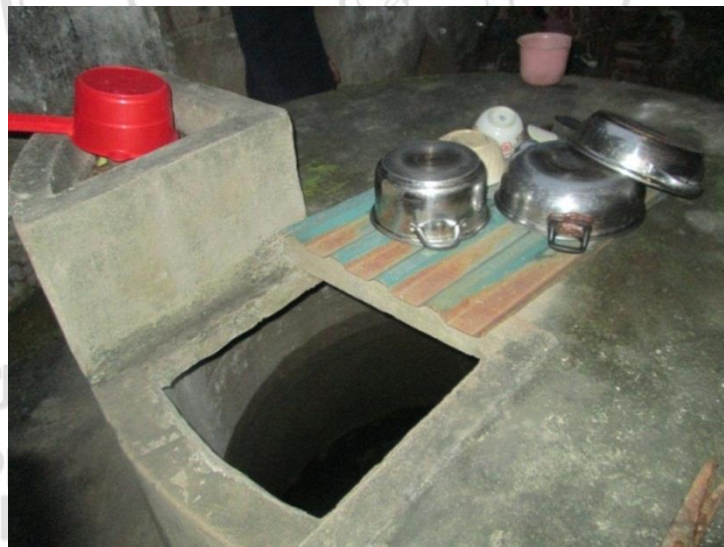
Figure 3.5 Water tank for rain accumulation
