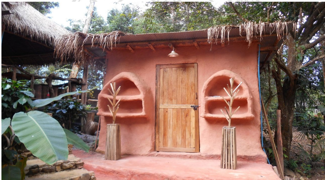
Figure 4.55 Local Materials in homestay (Taken on 18-11-2015 by Pradip)
