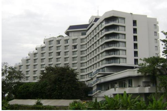
Figure 4.2 Concrete shear Wall (C2)
