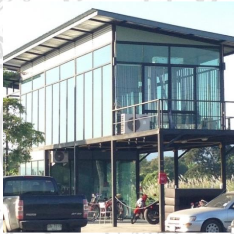
Figure 4.6 Light metal frame (S3)
