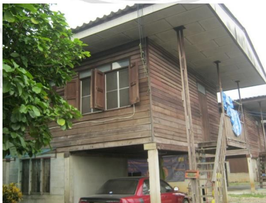
Figure 4.10 Concrete frames with unreinforced masonry infill with light wood frame building, Area \leq 464.5 sq.m. (W1C3)
