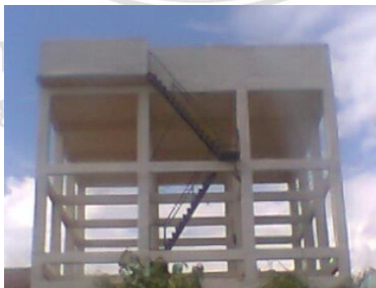
Figure 4.1 Concrete moment resisting frame (C1)
