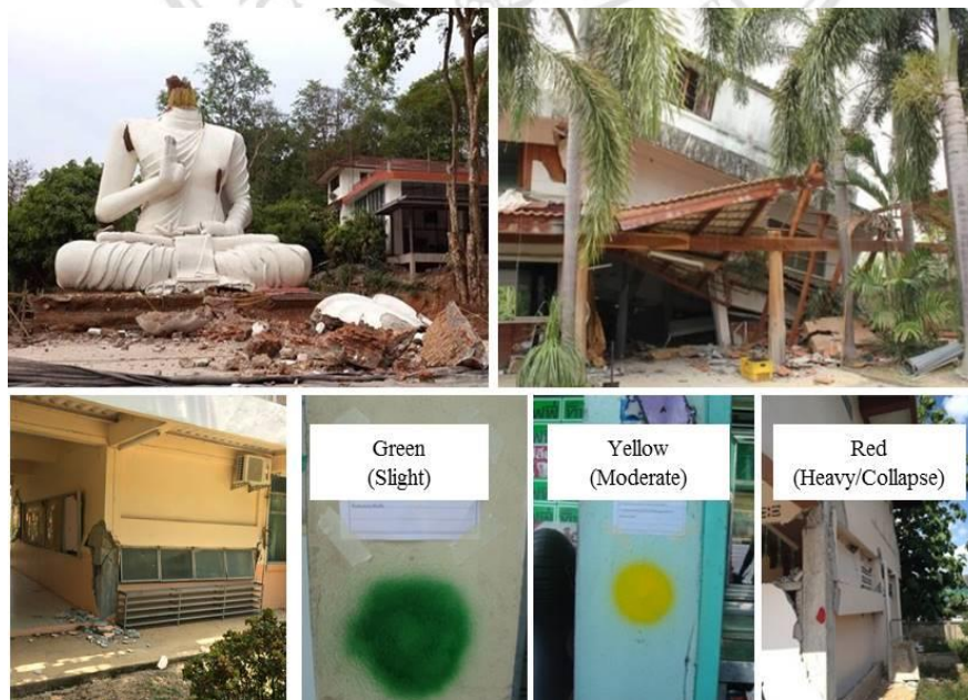
Figure 5.8 Building damage levels (Green, Yellow, Red with paint-sign), categorize by Department of Public Works and Town & Country Planning, Thailand
