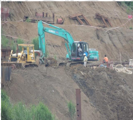
Figure 4.17 Men Working at Paletwa Jetty
