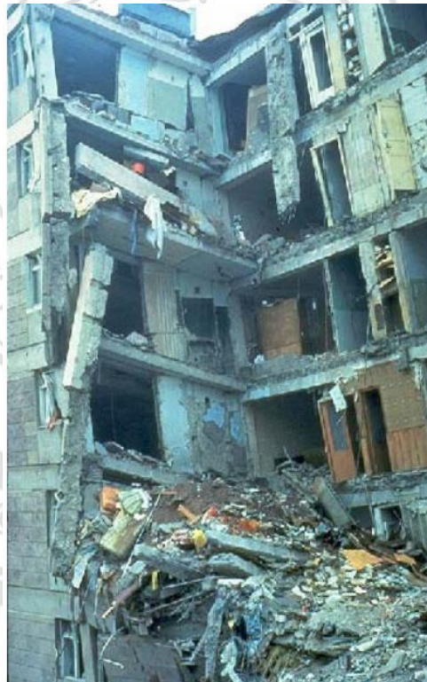
(c) Damage to 9-story precast concrete frame-panel apartment building in Leninakan ( http://www.hellerjohnsen.com/Spitak,%20Armenia%2012-7-88.pdf )
