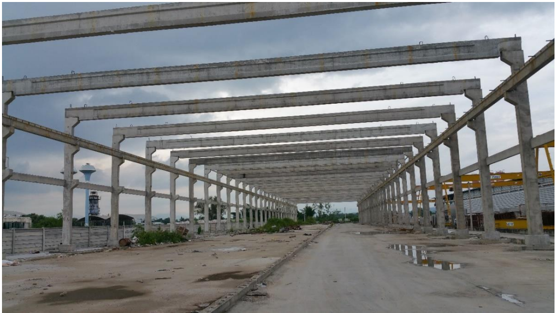
(a) Precast concrete construction for factory building
