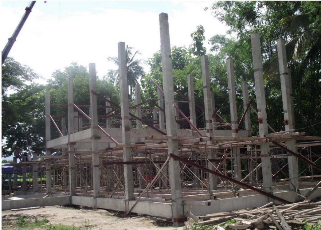
(c) Precast construction for residential building
