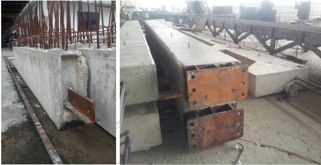
(a) Precast beam element (b) Precast column element with steel socket
