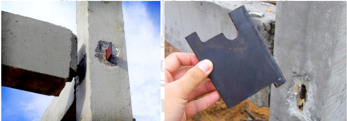
(a) Beam-to-column connection with sliding plate
