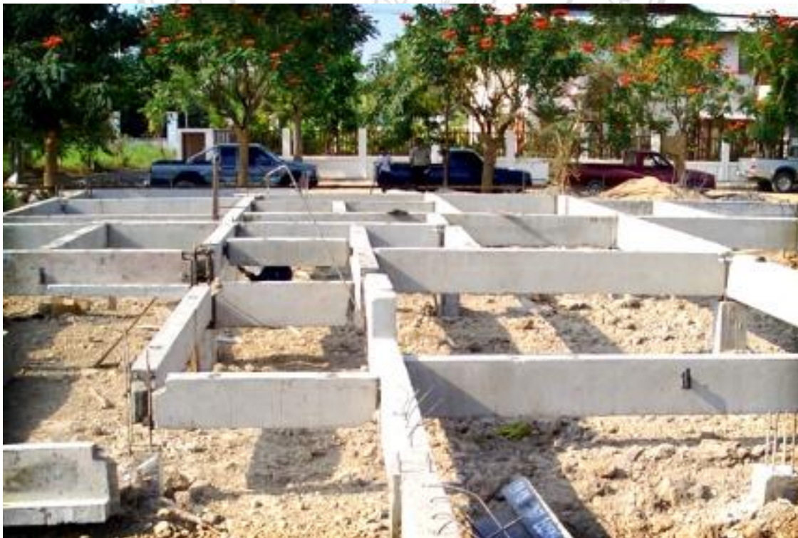
(b) Precast concrete construction for residential building
