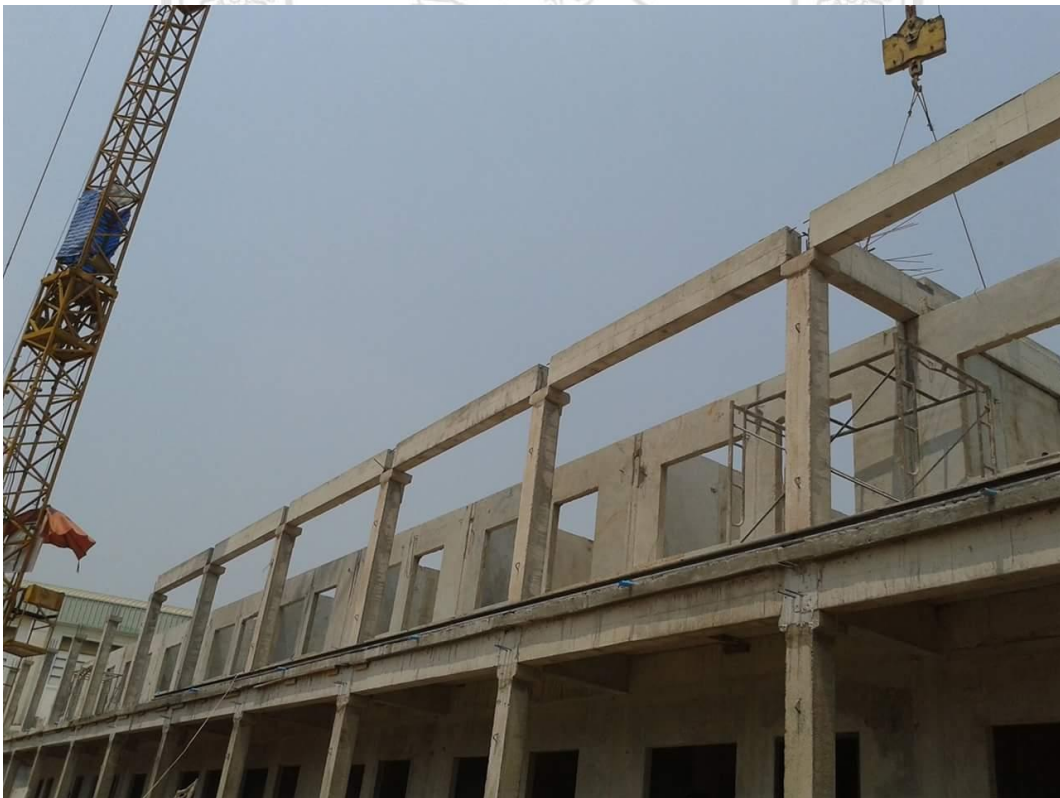
(b) Installing process for multi-storey concrete building ( https://www.facebook.com/Precast-Khon-Kaen/ )
