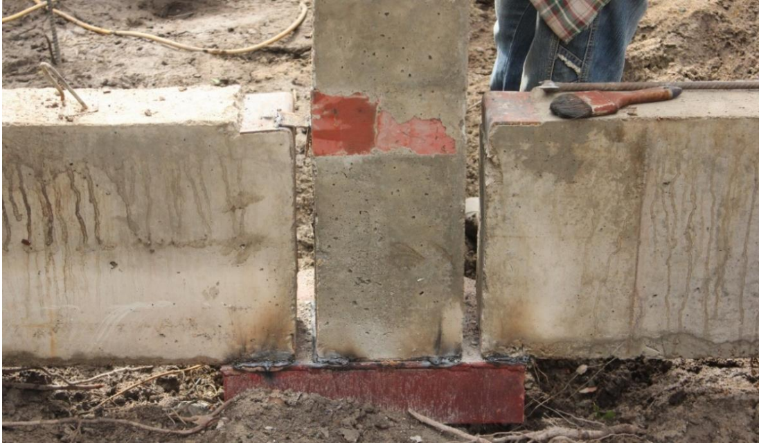
(a) Welding type of precast connection
