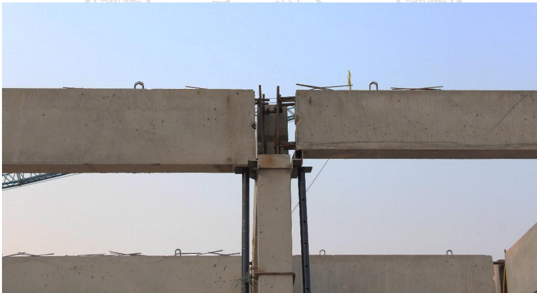
(b) Precast beam-column connection
