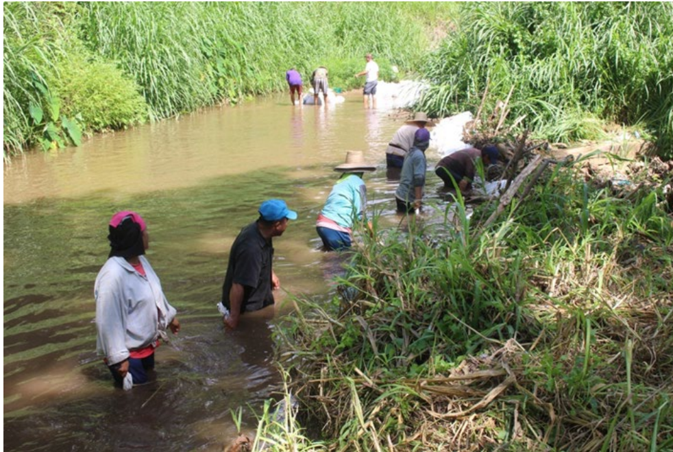
Figure 3.23 Local farmers piling up sandbags as weir to direct water to their rice fields during the cultivation season
