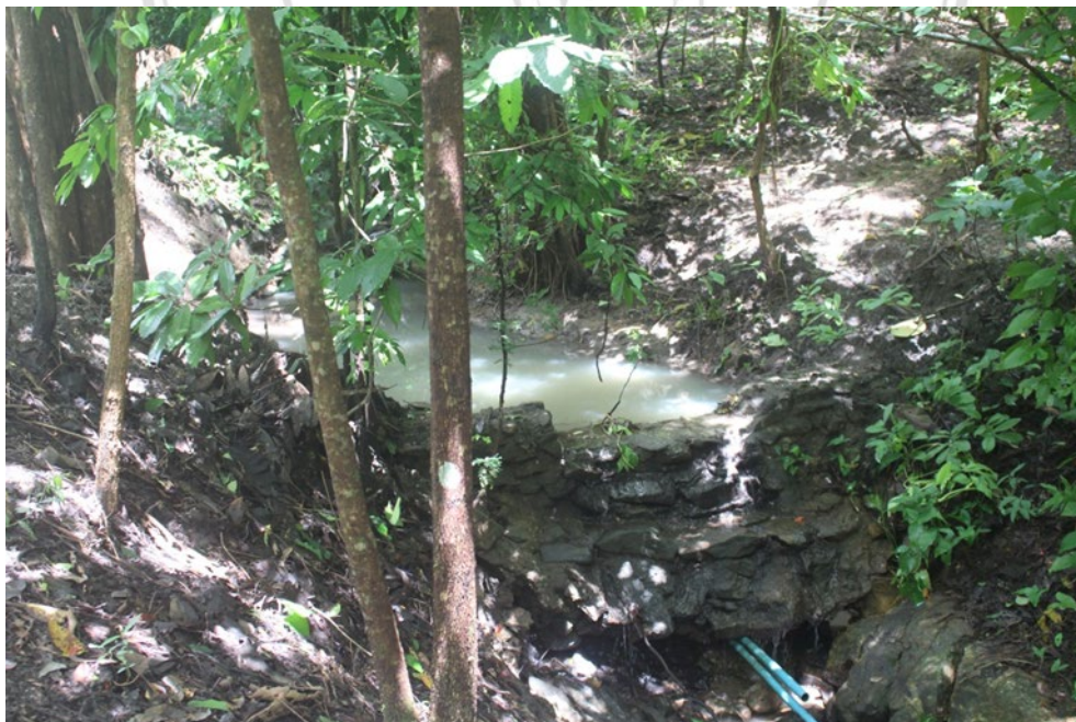
Figure 3.32 Water retention by rock weir after dredging, and the capability of slowing down water current of minor stream on slope
