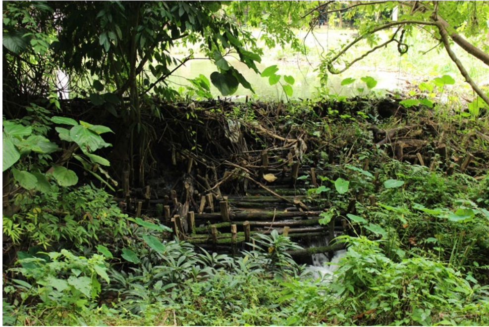
Figure 3.2 Hardwood Fai to Block Water Stream, with Cores Held Together with Crossed Wood Sticks
