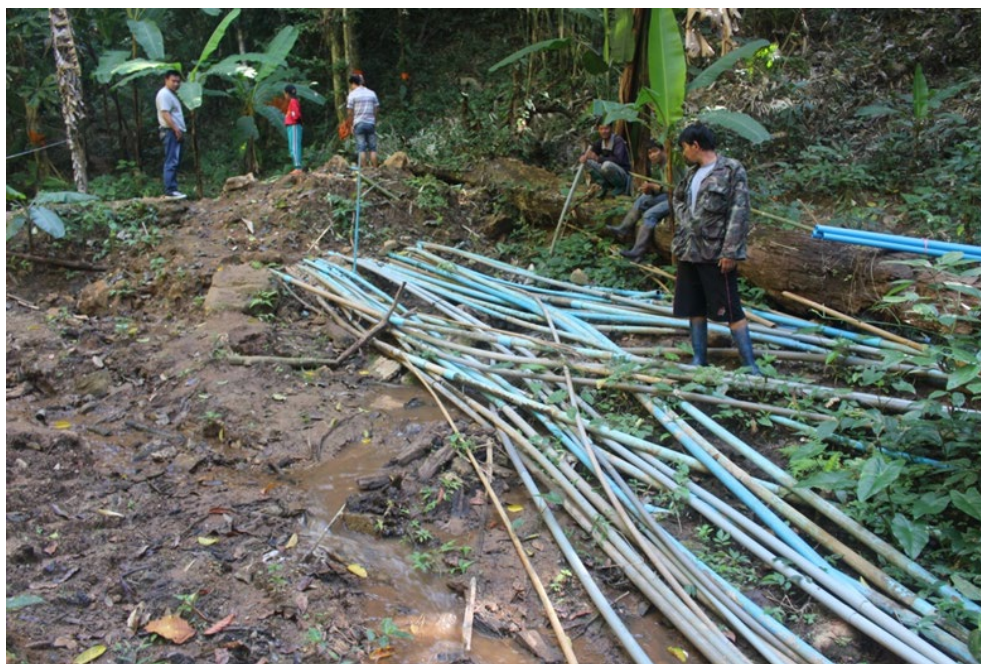
Figure 3.25 The use of pipelines to direct water from the spring, there are a great number of pipelines in different sizes which reflect the absence of the agreements on water use, which is a cause of water shortage during a dry season
