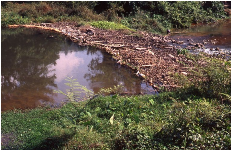
Figure 3.1 Bamboo Fai to Direct Water to Agricultural Fields in Village Level
