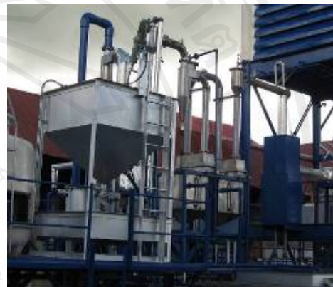
ง. Flocculation Tank
