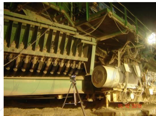
Transfer point Line N
