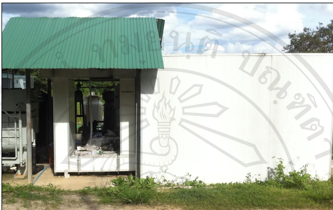
Figure 2.7 Side view of the testing room.
