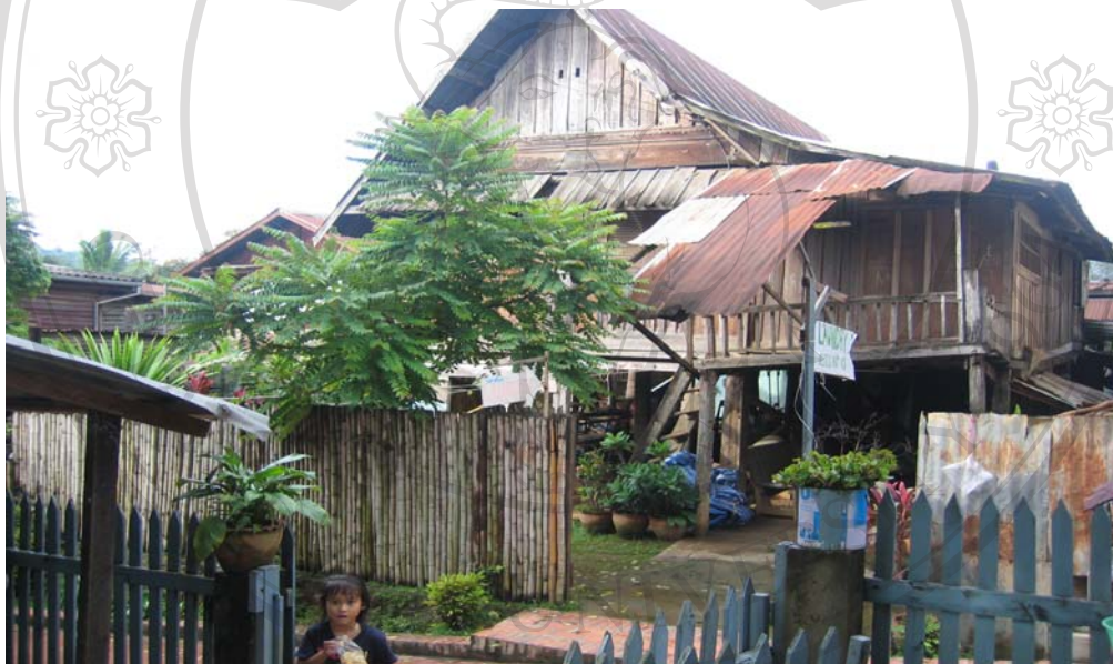
Figure 3.10 One of the Deteriorated, Listed Wooden Houses
