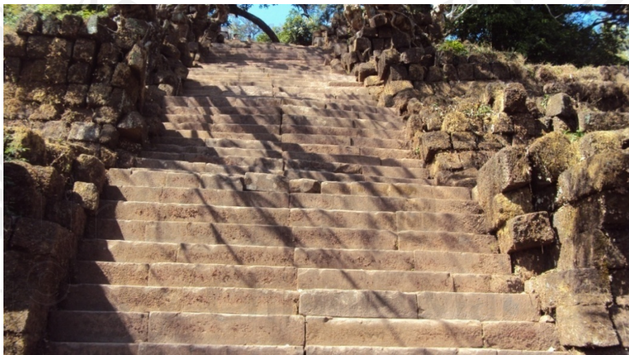
Figure 2.10: Staircase; Photo taken in December 2011
